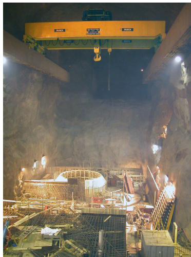
370t crane from Munck Cranes
