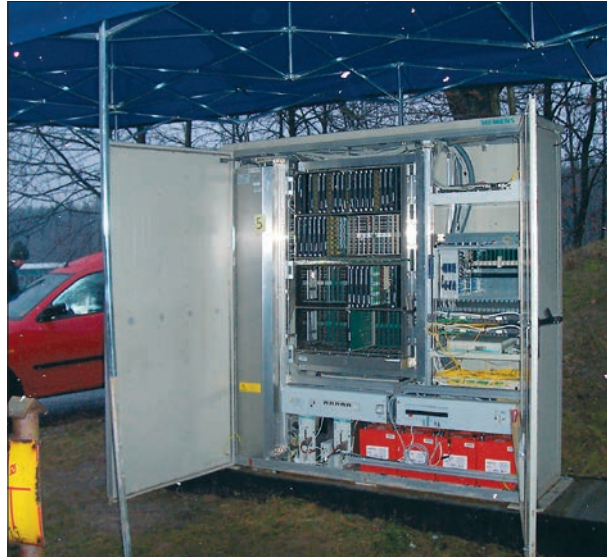
Cabinet before extension
