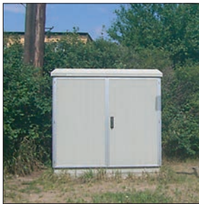
Cabinet before extension
